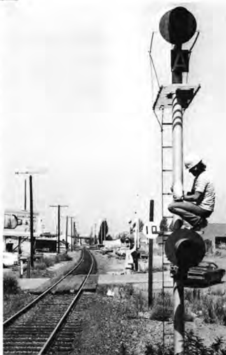
Signal Maintainer, Gary Patch, applies safety tape on signal pole on WP's main line near downtown Oakland.
