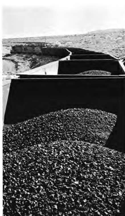
Ballast train awaits instructions for unloading.
