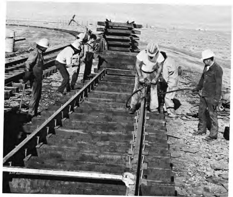
Foreman Ed Lowe and extra gang 205 man the track panel assembly line with the assistance of air powered tools. These men can assemble 24 panels per day or about one panel every 20 minutes.
