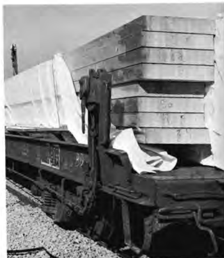
The roof trusses are made of laminated wood beams and shipped on 85 ft. flatcars to the construction site.
