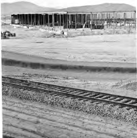
The roof trusses are made of laminated wood beams and shipped on 85 ft. flatcars to the construction site.
