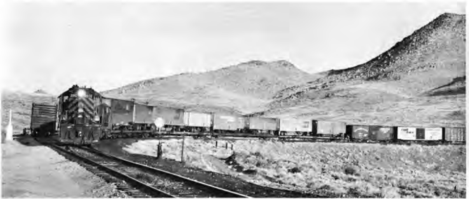
WP's Reno local provides daily early-morning piggyback and carload deliveries to Reno and North Reno industries.
