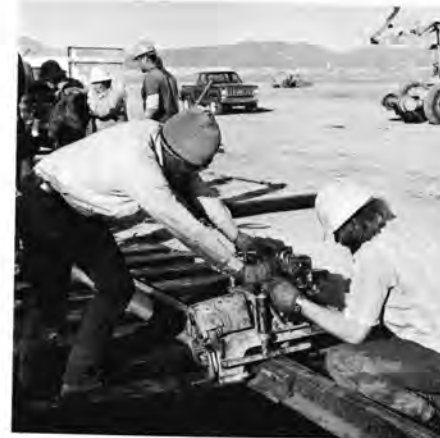
Track gangs install new joint bars (left) first using the drilling machine to make new bolt holes in rail and (right) using a bolt tightening machine.
