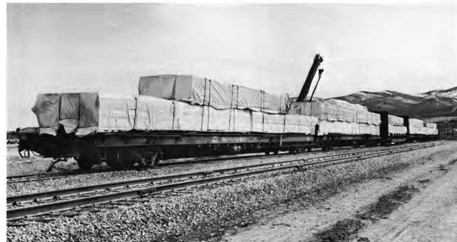
First commercial loads of building material are delivered to the siding. The materials include roof trusses for construction in the large new warehouse.
