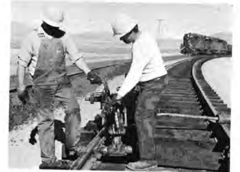
Track gangs install new joint bars (left) first using the drilling machine to make new bolt holes in rail and (right) using a bolt tightening machine.
