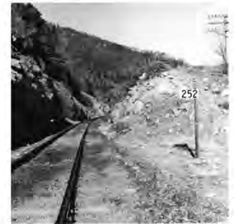
MILEPOST 252: Looking east, this picture is taken six-tenths of a mile west of the bridge at Tobin which crosses the Feather River and places the WP Main Line on the south side of the river.
