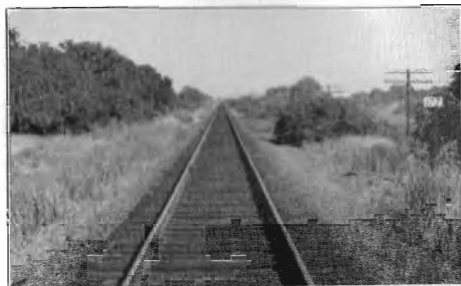
*Milepost No. 177: Straight ahead to Marysville about 1½ miles distant.
