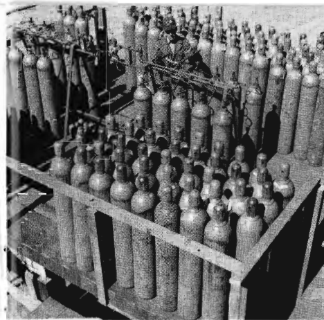
Oxygen tanks brought in by carload are connected to header pipes by David Mentaberry.
