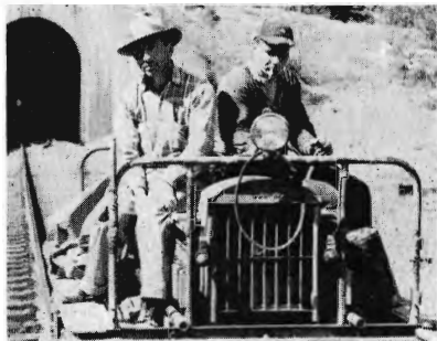
Roscoe Powers, foreman, Tunnel Gang 4, and Edward Wells, B&B carpenter, outside Tunnel 1, near Niles.
