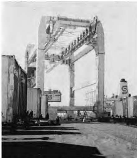
One of two sliding boom 45-ton cap. mobile cranes which run along 700'-long pier.
