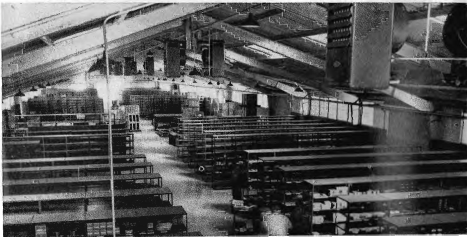
Interior view of the 320-foot long new store building, taken from the roof of the store building office. Building is air-conditioned, roomy, and well lighted. The stock is now being transferred to new shelves.
