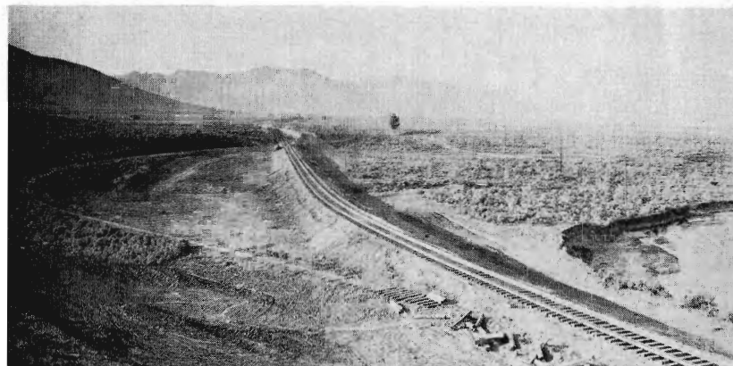
WP's new line straightened out many NCO curves.
