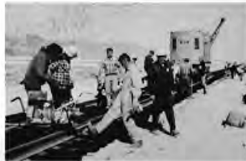
Above and right: Nearly 37,000 treated ties and more than 69,000 track feet of rail were used in construction of the new branch line.
