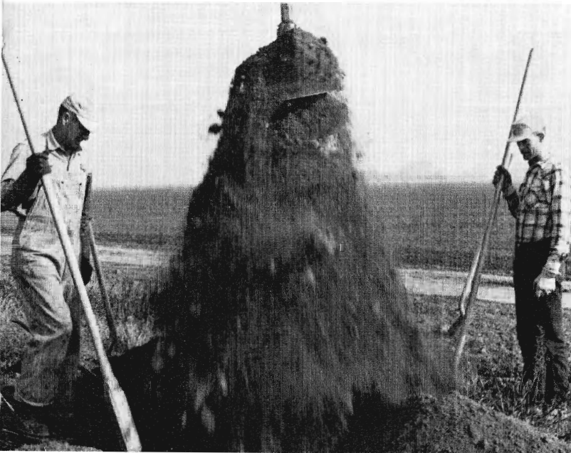
Below: Pushing another lever on the truck's control panel, Hurley puts the auger into a little rock 'n roll and twist, shaking loose load of dirt which will be tamped around anchor.
