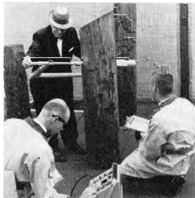
Engineers developing work on nuclear equipment to determine piling and timber decay.
