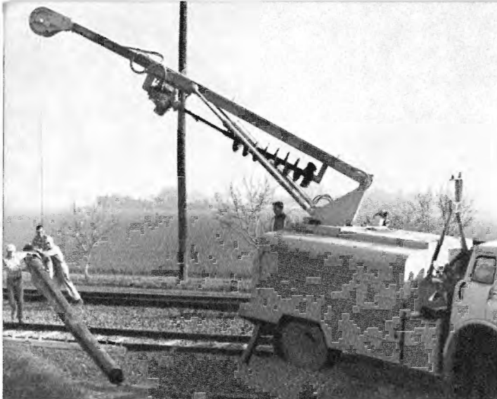
Left: Easing a long pole up through existing wires is a tricky job, requiring skill and careful handling by crew (not all visible), and truck, but job was completed without a hitch.
