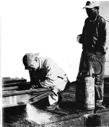
When welded rail leaves the Winnemucca welding plant each end is tapered so that it will slide easily on and off the cars. Welder C. W. Wilkins cuts off one end while Helper Raymond S. Gonzales stands ready with tank of water to extinguish any fire caused by flying sparks. The rails were then cut into lengths required for the job as previously marked by the engineering party shown on this month's cover.
