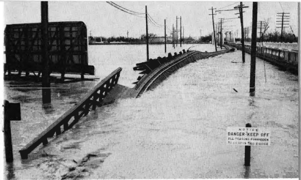
The Sacramento Northern trestle began twisting from the force of the Feather River about 1 p. m., December 23. Later that night the entire span washed away, as did a section of the Fifth Street Bridge, right. Photo, looking west from Marysville, by Robert Hardy, Marysville Appeal-Democrat . Below, C. C. Cox's camera looks east towards Marysville, same location.
