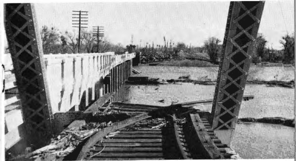
The Sacramento Northern trestle began twisting from the force of the Feather River about 1 p. m., December 23. Later that night the entire span washed away, as did a section of the Fifth Street Bridge, right. Photo, looking west from Marysville, by Robert Hardy, Marysville Appeal-Democrat . Below, C. C. Cox's camera looks east towards Marysville, same location.
