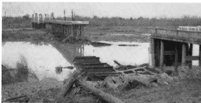
Looking west across the Feather River towards Yuba City, picture shows washed-out Sacramento Northern tracks, lower center, which crossed river alongside of the Fifth Street Bridge.
