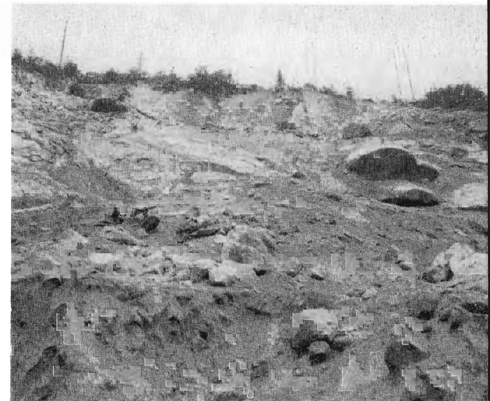
Looking up the upper face of the slide, huge boulders dwarf the tiny-appearing bulldozer and operator pushing away, shovelful after shovelful, tons of dirt and rock.
