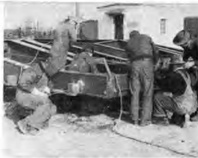
Welding parts to underframes.
