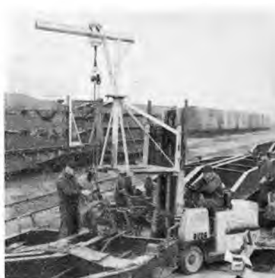
A swing boom jib crane was built for use with a fork lift truck to handle heavy items such as draft gears.
