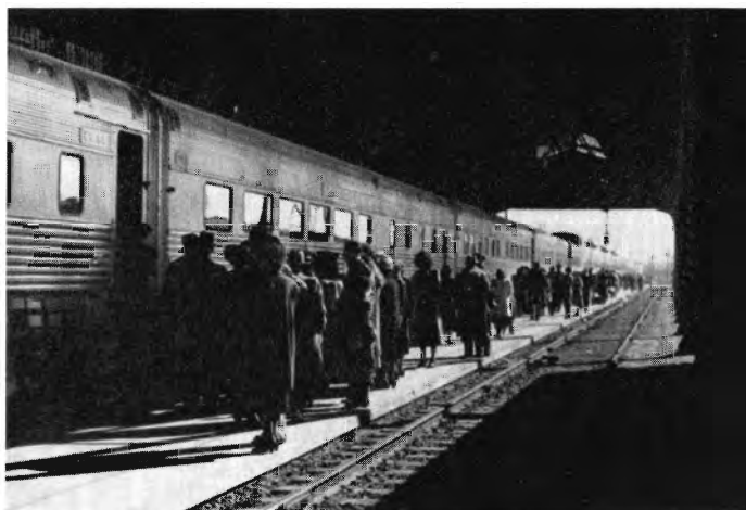
The eastbound California Zephyr on July 29 was the last WP train to leave Oakland Pier's trainshed.
