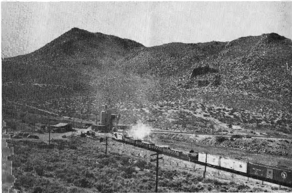
A Reno local waits just outside the east portal of Tunnel 37 for clearance to pass through on way to Portola. Temporary cement plant is shown at junction of Reno Branch and WP's main line. Old shoo-fly roadbed may be seen midway up mountain on left, just below thin white line of high tension power line.
