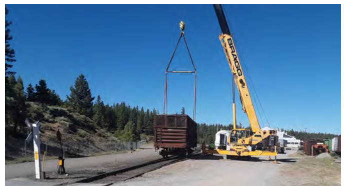
Almost a year after the proposal to donate one of our beet gondolas to the Arizona Railroad Museum was approved at the July 2018 FRRS Board Meeting, SP Beet Gondola SP 359247 is being loaded leaving the WPRM for Arizona.
