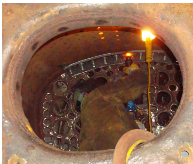
Norman riveting into the knuckle patch.
